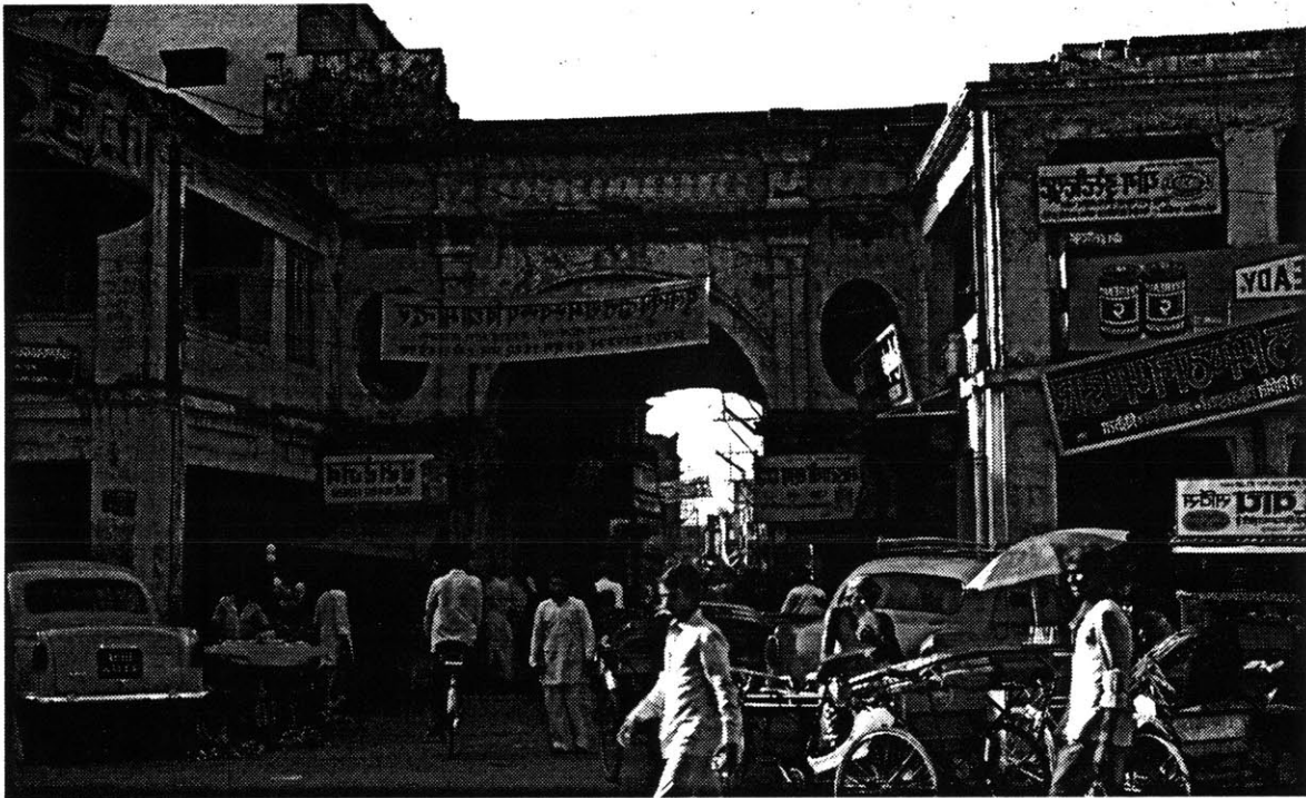
Figure 55: View of Entrance to Chauk.
