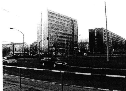
Fig. 4.30 - Tower structures in the Seevorstadt West district.
