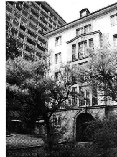
Fig. 2.25 - Photo showing the entry into the courtyard and stairwell to apartments.
