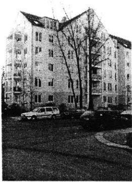
Fig. 5.26 - Renovation, Seevorstadt East
