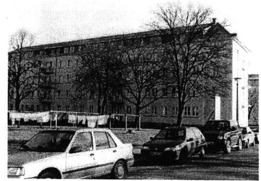
Fig. 5.20 - Expanded attic space, Johannstadt
