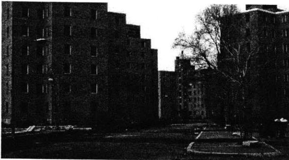
Fig. 5.6 - Existing street view of the Columbia Point project.
