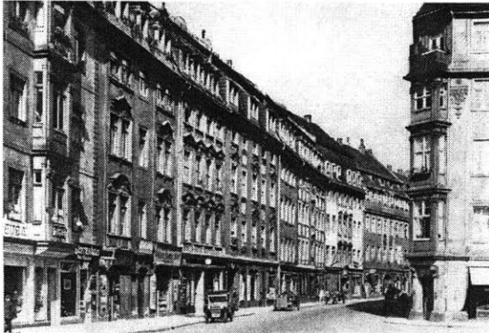
Fig. 2.8 - Urban housing that creates a uniform street with distinct horizontal subdivisions.
