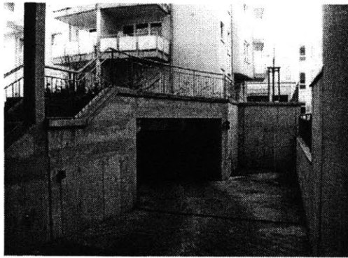
Fig. 5.24 - Underground Parking, Seevorstadt West
