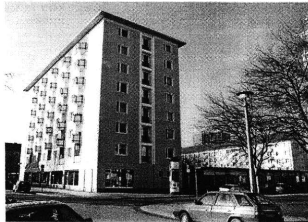
Fig. 4.31 - Tower structure in the Seevorstadt East district.
