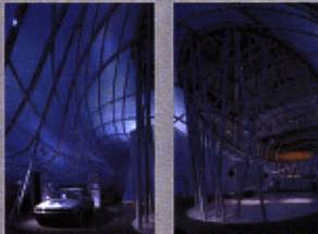
The BMW pavilion uses CAD/CAM technologies to create two organic forms of water droplets with conventional steel ribs as structure.
