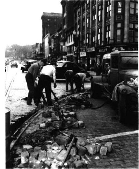
Fig 2.11 Trolley tracks being installed along State Street near Broadway in Schenectady.
