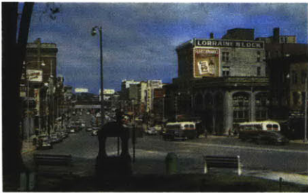
Fig 7.13 View from Veterans Park towards Lorraine Block.
