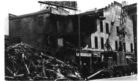
Fig 7.11 Demolition of the Ellis Building
