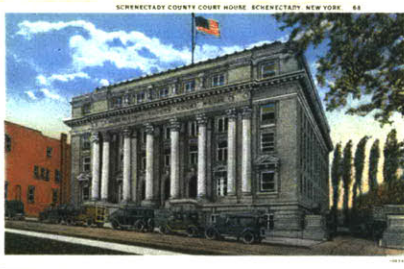
Fig 9.17 Courthouse across Veteran's Park from MVP.
