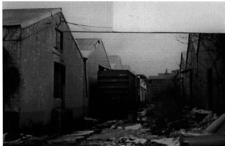
Fig.4.3 Warehouses and train-spurs on the site. The new Museum of Industry and Science Park will reinterpret these left-over constructs, celebrate them, all-the-while teaching visitors of an important New England history.
