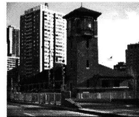
Fig. 4.5 The old Charles River Dam support buildings contain massive engine-powered, sliding water-lock doors. These structures should be preserved and celebrated as a part of the Science Park.
