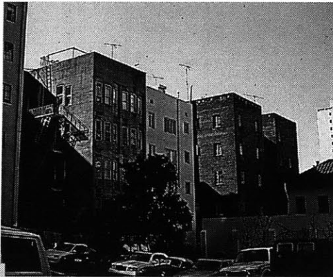
fig.25 View of surrounding buildings on the west boundary of the site
