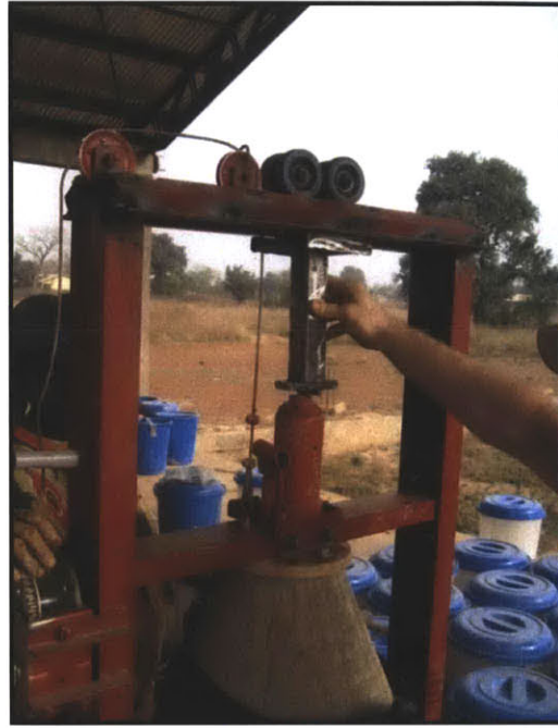
Figure 4-8: Sliding the jack into place
