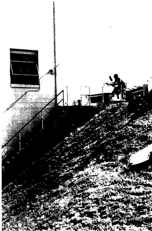
Site Photo, levee at pump station
