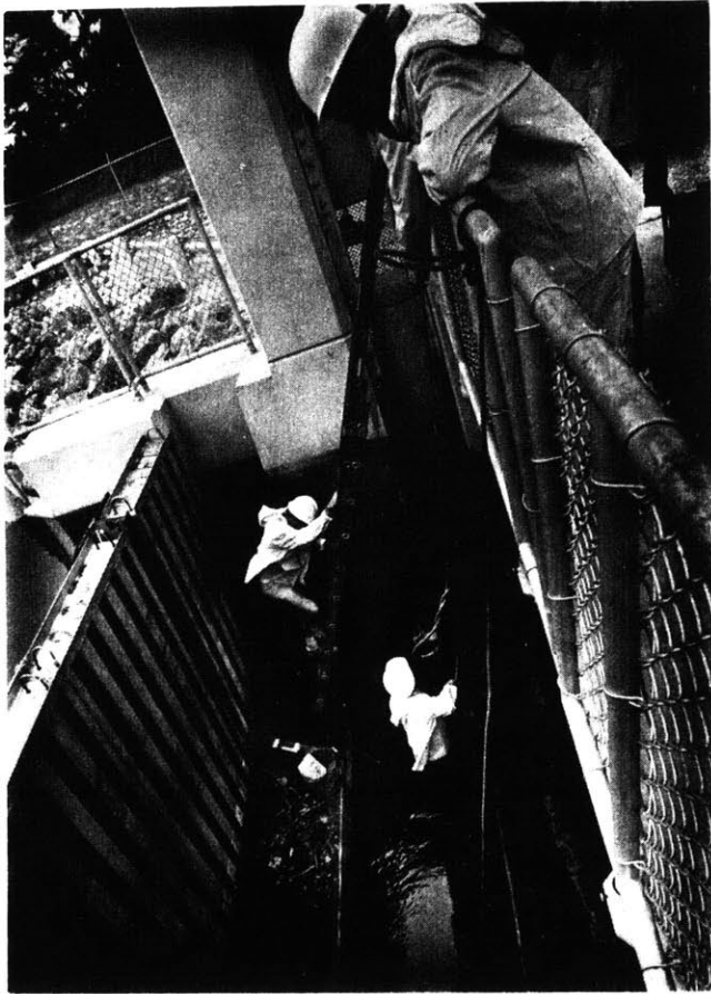
Climbing into a spillway
