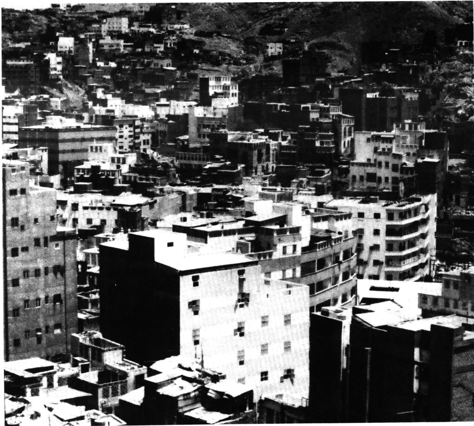
An overview of Al-Garara locality, where traditional houses are being demolished and replaced with "modern" high rise buildings.
