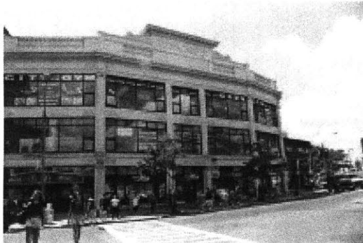
figure 19 view of intersection of Brookline and Commonwealth Avenues
