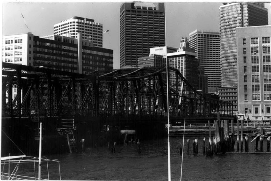
Northern Avenue Bridge.
