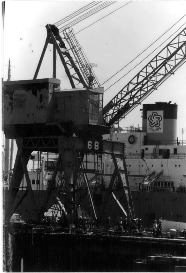
Crane in operation at South Boston Navy Yard site
