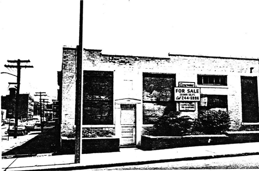
Clearwater Laundry on Amory Street
