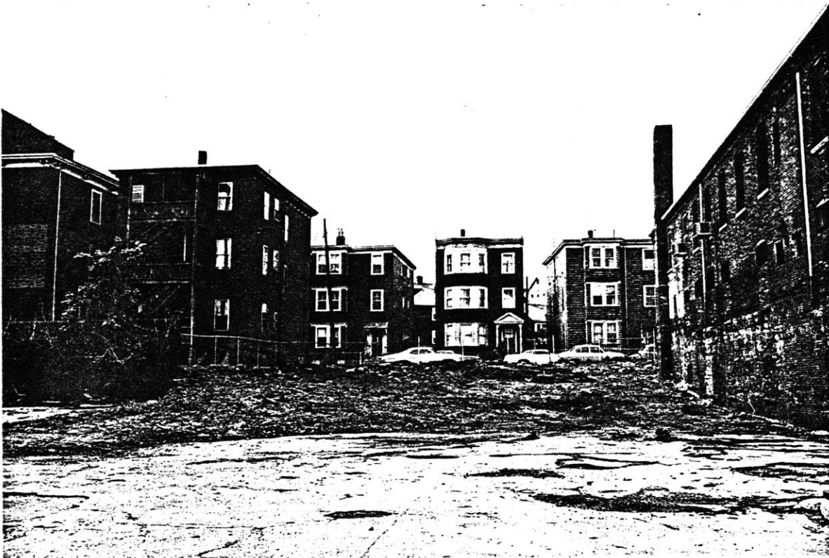
View toward Chestnut Avenue alongside Hammond's warehouse
