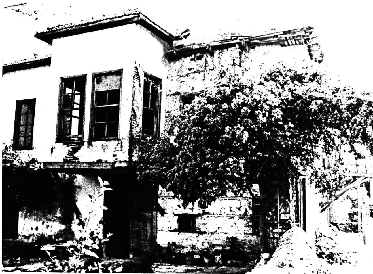
MAIN ENTRANCE - EAST -
