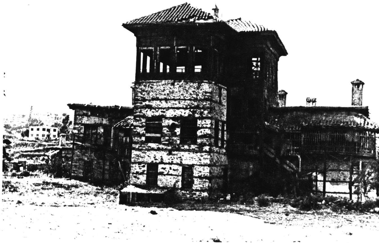
SOUTH EAST FACADE
