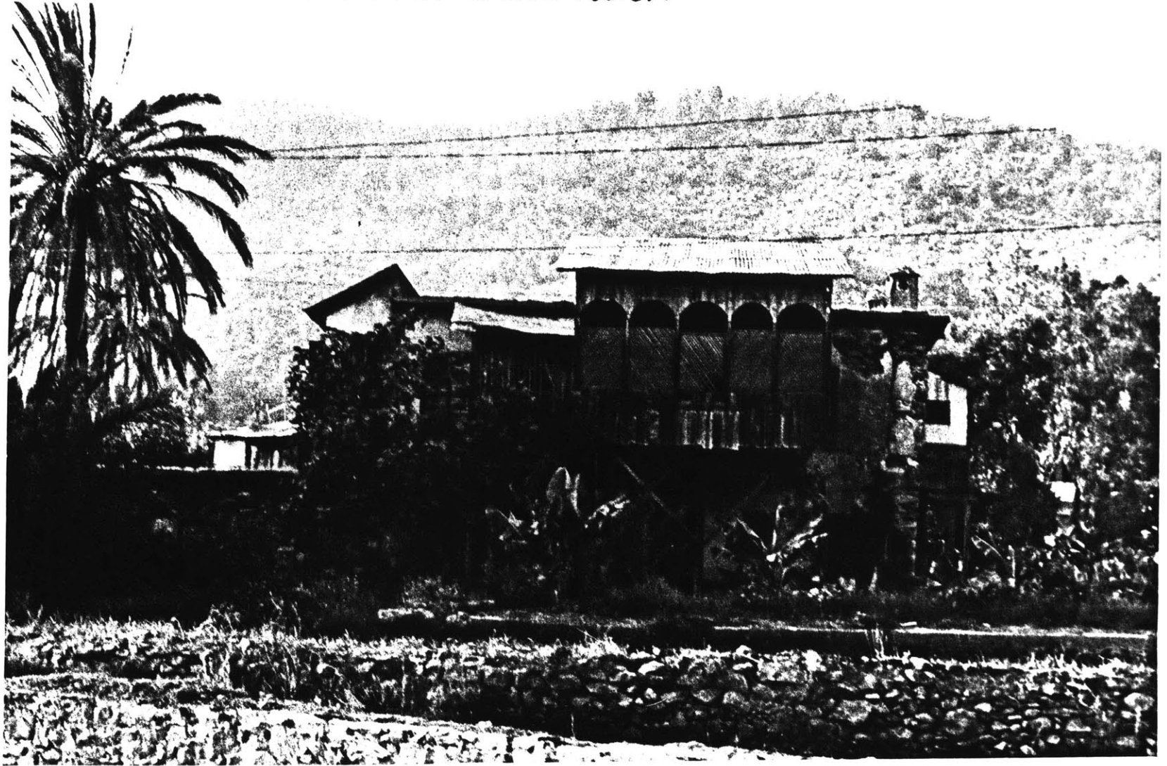
HOUSE. 7. HOUSE OF APTULLAH SABRI TÜZÜN
