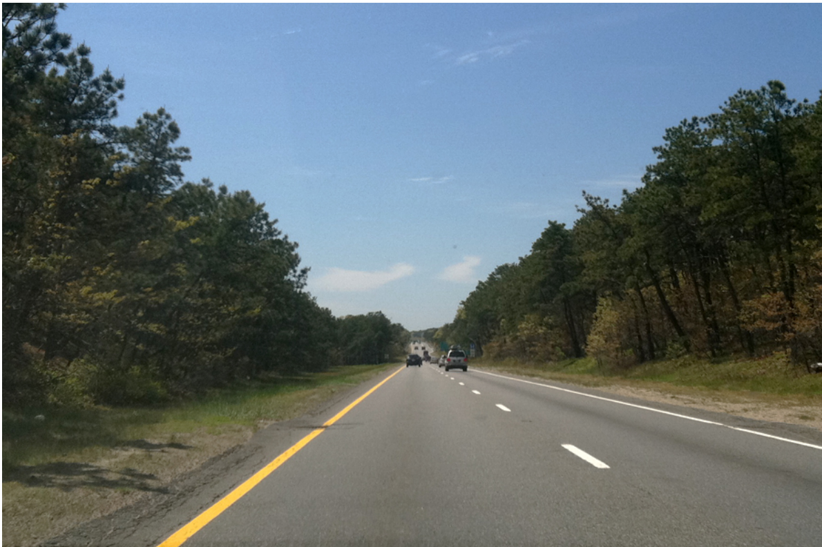
Figure 23. Massachusetts Route 6 (May 2012).
