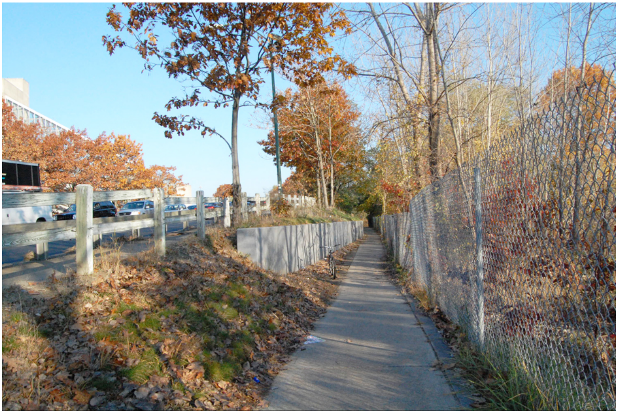
Figure 21. Ramp diverting bike and foot traffic from Route 2 (October 2011).
