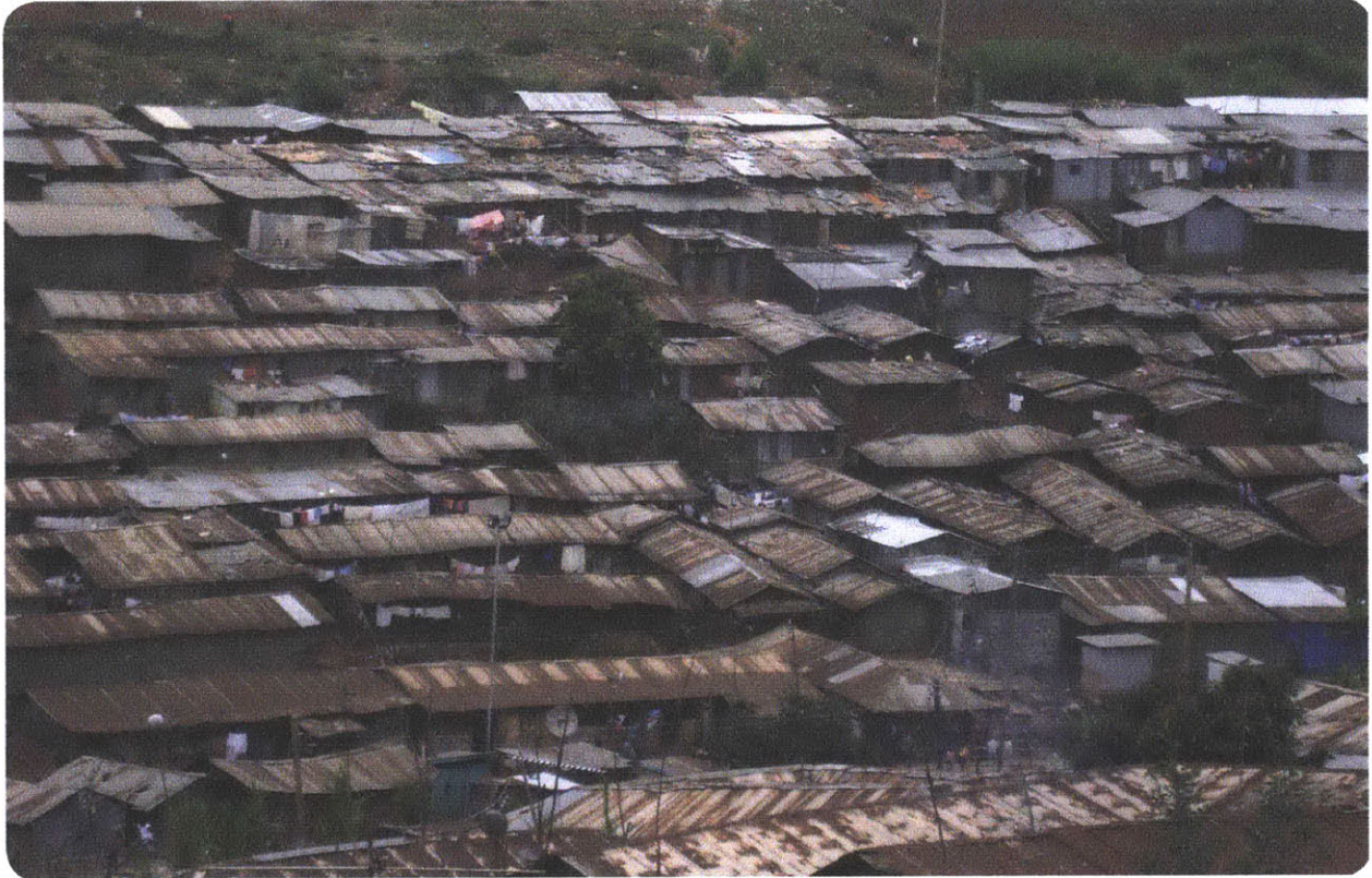
Site Image of Settlement Rooftops
