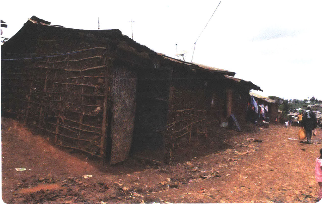
Site Image of Wattle and Daub (Mud) Construction
