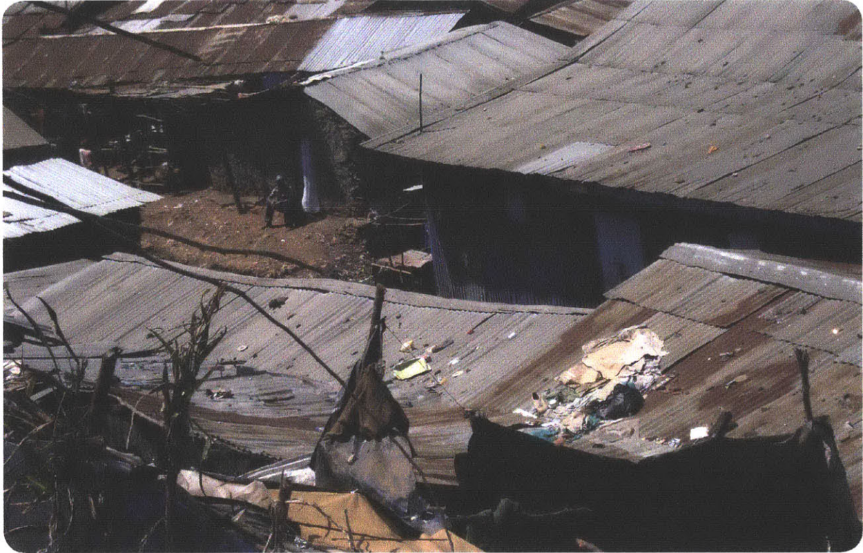
Site Image of Corrugated Metal on Bush Pole Structures
