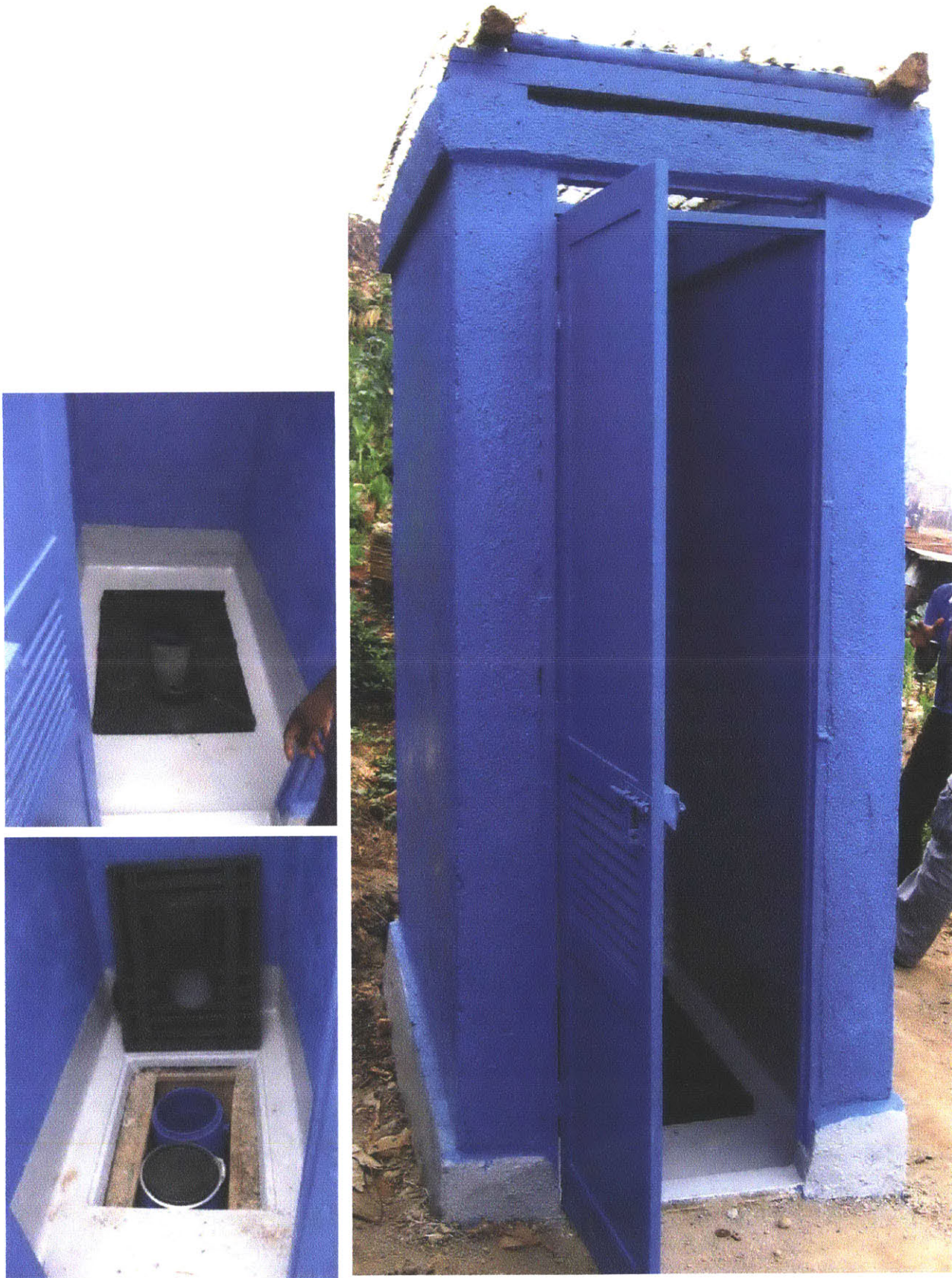
Photos of Eco-San toilet in operation on Kibera site, Summer 2010
