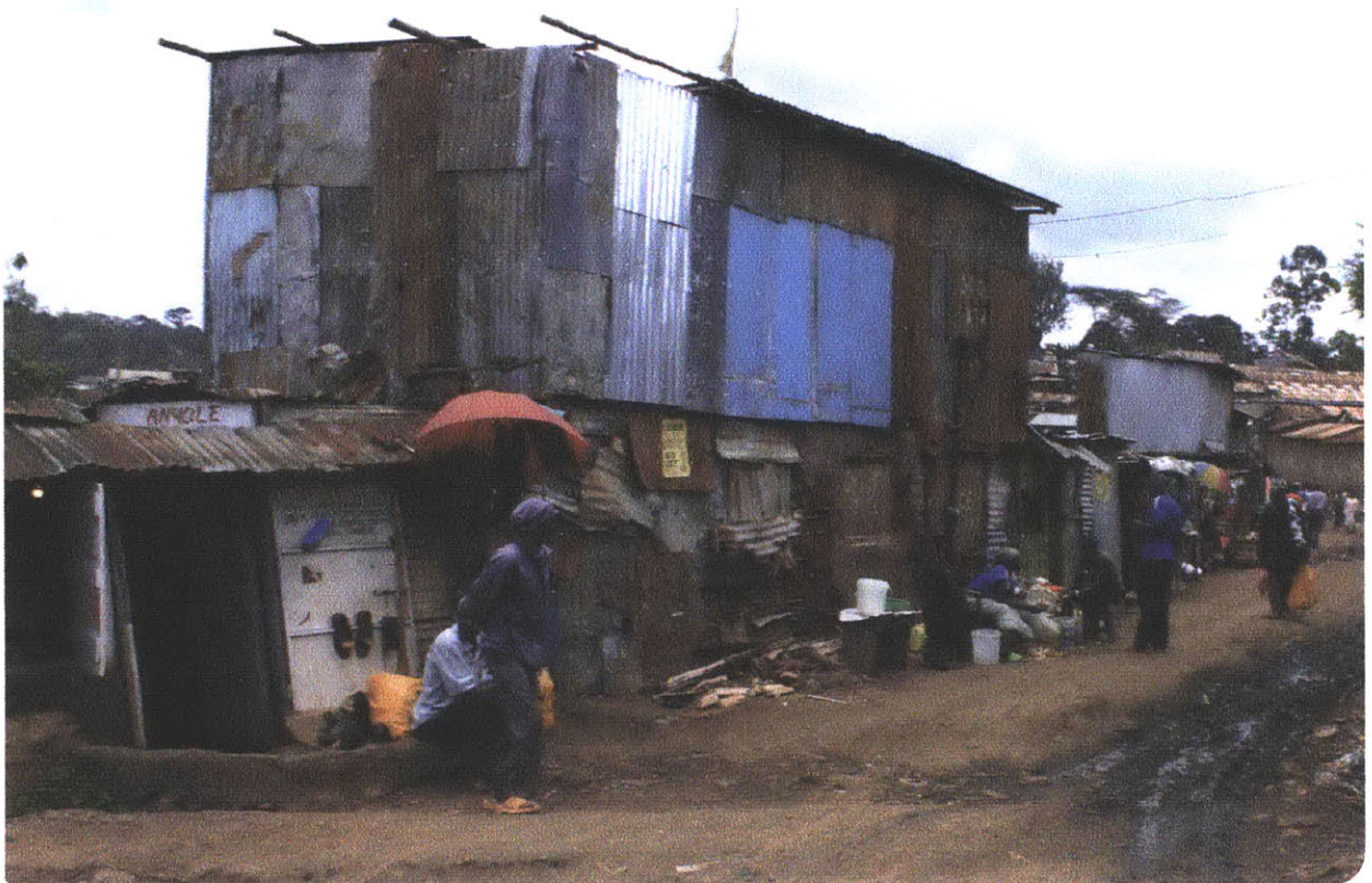
Site Image of Corrugated Metal (Iron) Sheet Construction
