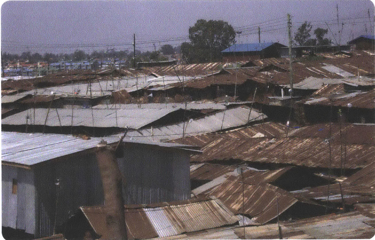
Site Image of Rooftop Antennae
