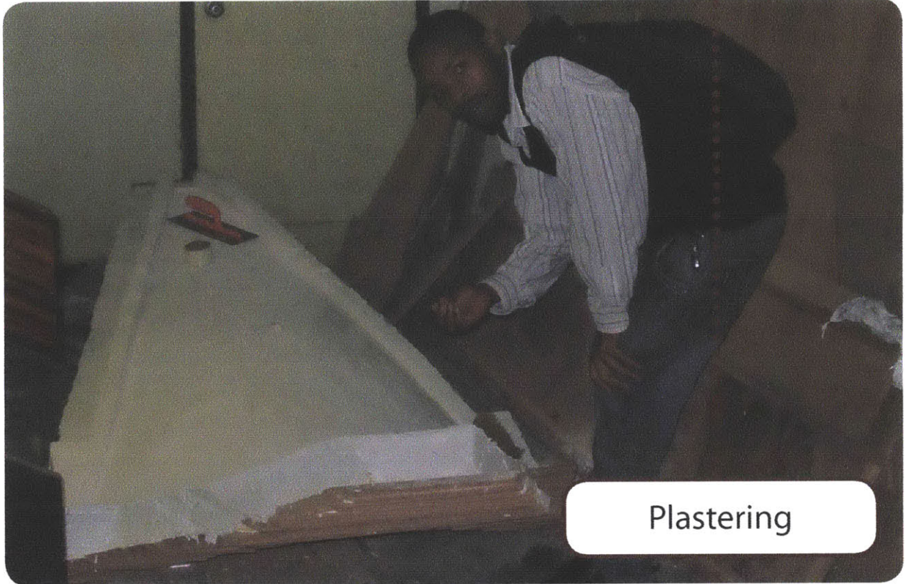
Dec 1st | Plaster was slow to dry due to rainy weather
