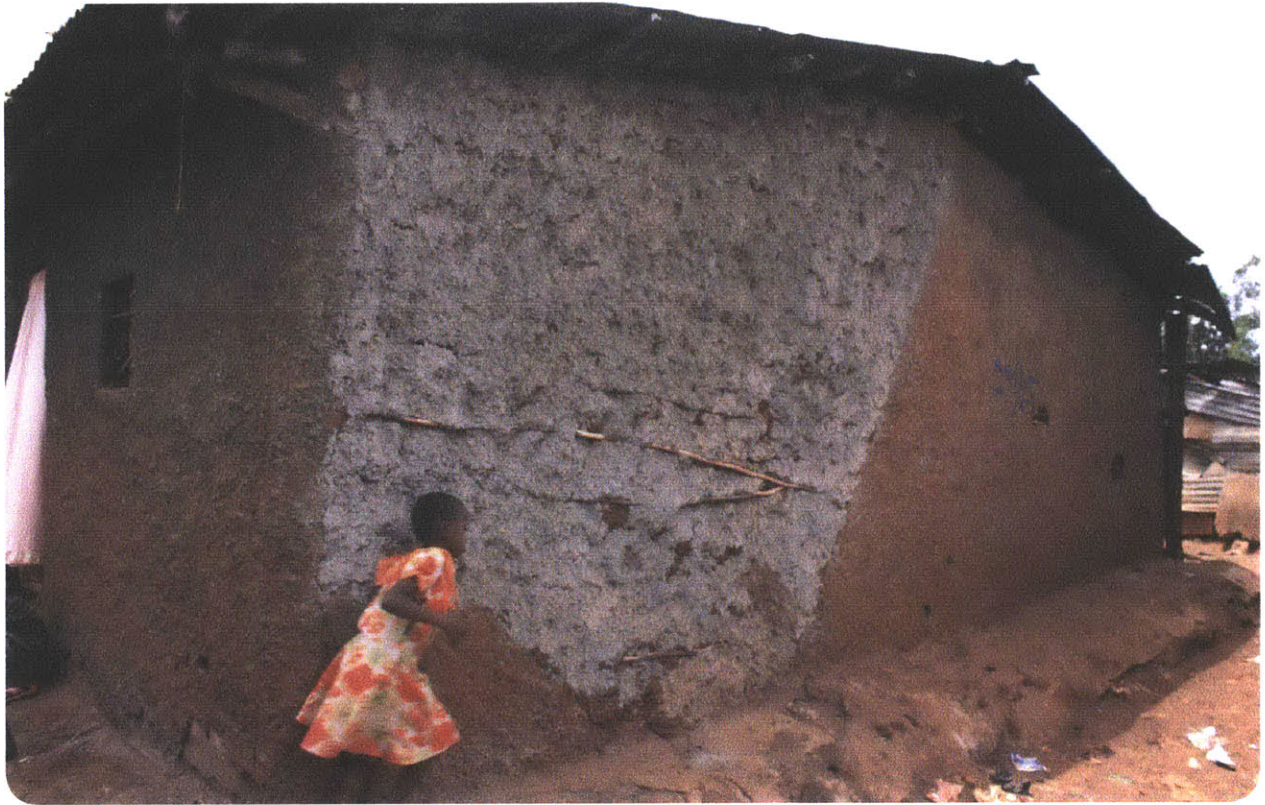
Site Image of Cementous Plaster on Mud Construction
