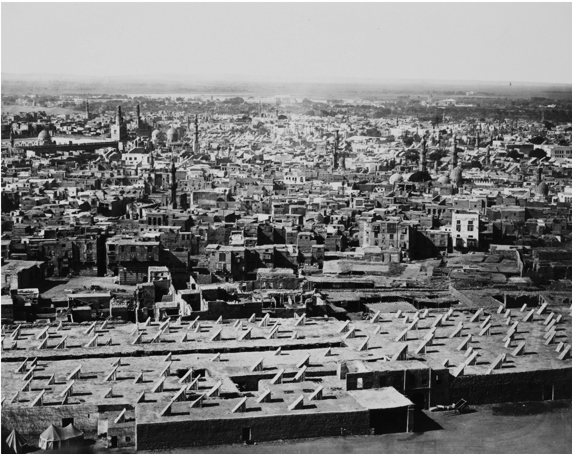
Figure 1-3: Photograph of Cairo from atop the Citadel, 1860. Photo by Frith (20). A close inspection shows the abundance of windscoops across the roofs of the city
