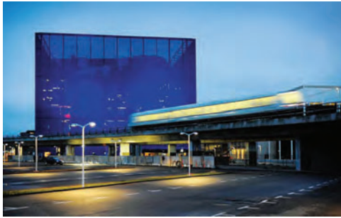
▲ Figure 41: Photo of the Danish Broadcasting Corporation Headquarters at Ørestad Nord ( Copenhagen Growing , http://www.orestad.dk/~media/Orestad/pdf/Copenhagen-Growing_web.ashx ).
