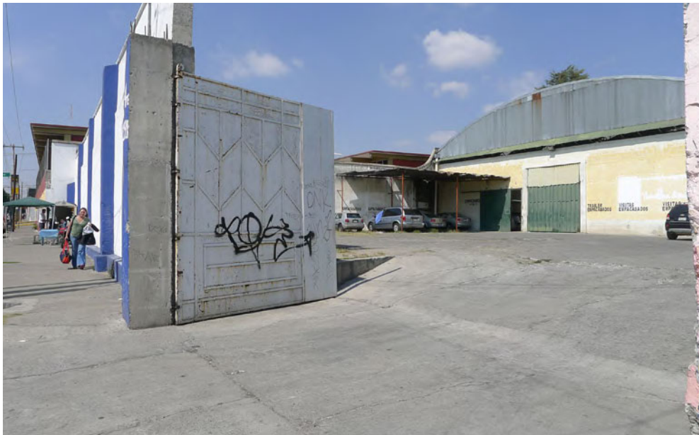
▲ Figure 87: Photo of industrial shed in the study area selected for Ciudad del Diseño proposal (by author).
