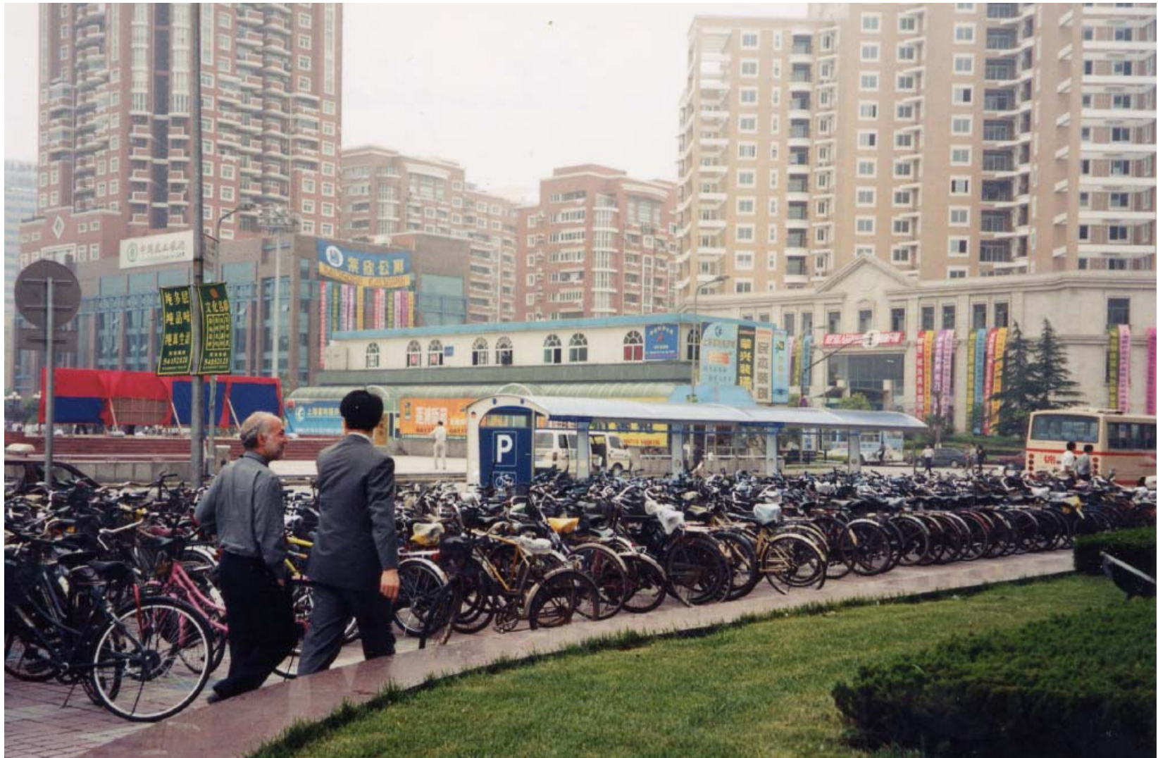
New residential/commercial construction in Shanghai and bike park
