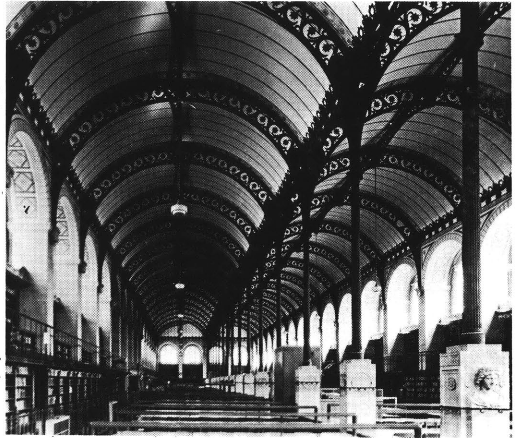
45. Austin, interior view.
