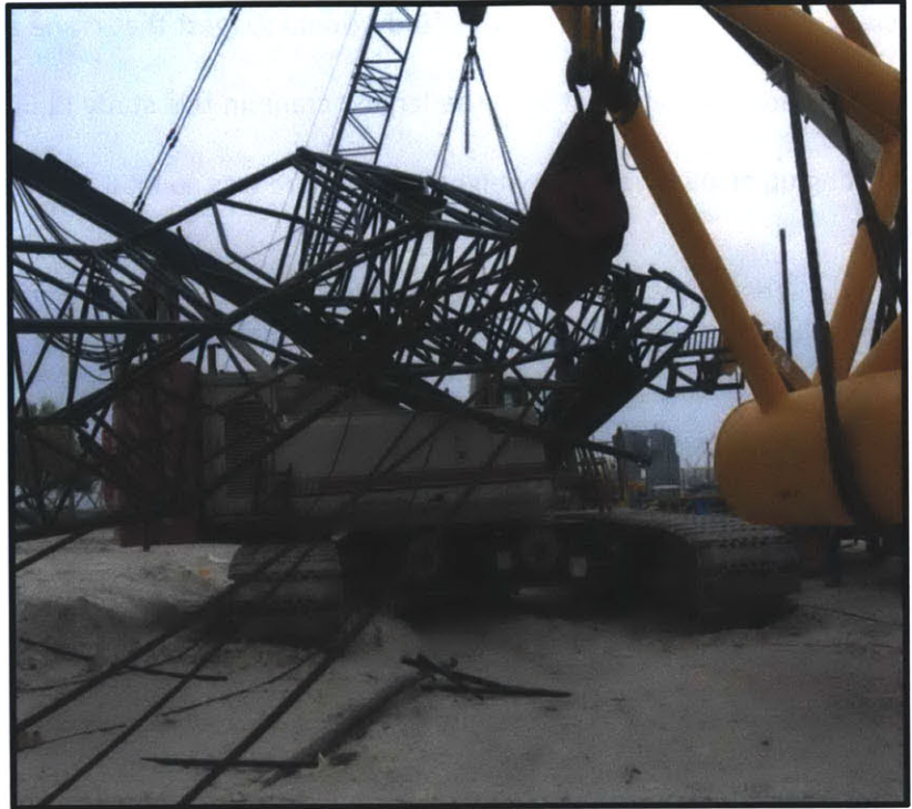
Figure 5.1: A collapsed lattice boom. Categorized as a “physical issue.” (Haag Engineering Co.)
