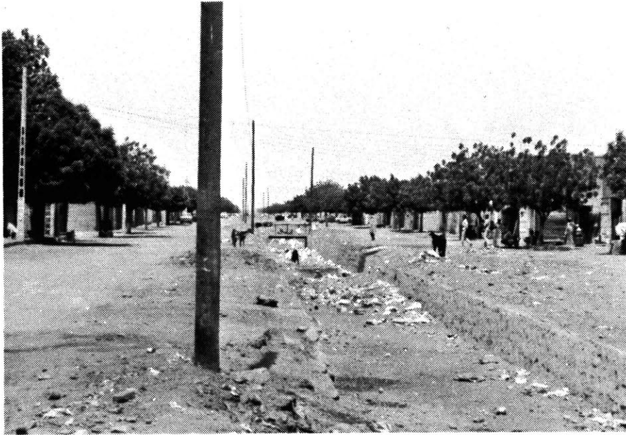
Photo 16: Al-Mahdiyya. When Left Open, Main Drainage Ditches Form Physical Barriers Between Dwellings, and Act as Dumps.
