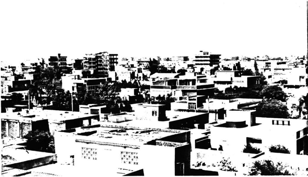
Photo 10: Al-Riyadh. General View.
