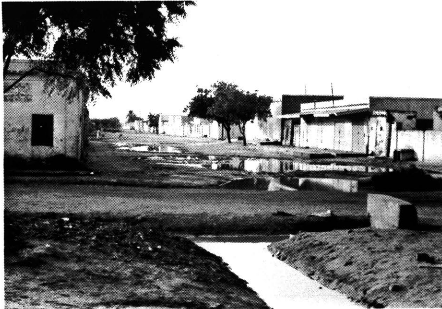
Photo 2: ...in a Residential Street Demonstrates the Inadequacy of Maintaining the Discharge System in the City.
