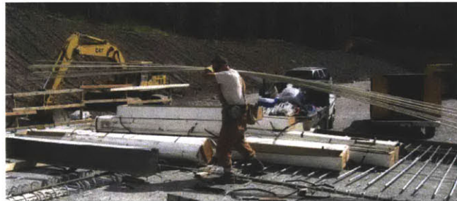
Figure 10: Carrying a bundle of FRP Rebar (Bisby 12)
