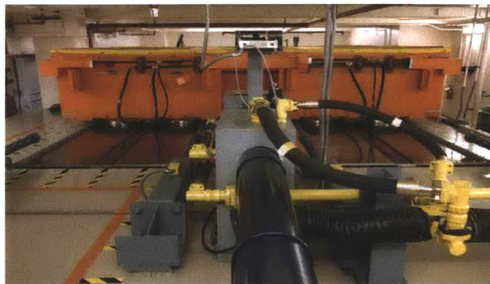
**Figure 16: Sliding TMD in John Hancock Tower [51]**
