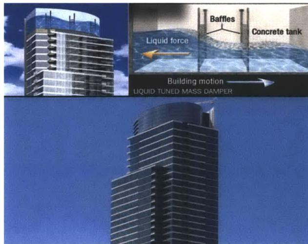
Figure 17: TLD in One Rincon Hill Tower in San Francisco, USA [40]
