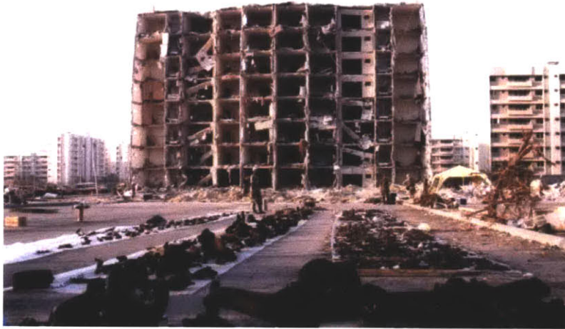
Figure 3.2: Khobar Towers BLDG 131 Damage (Source: DefenseImagery.mil)
