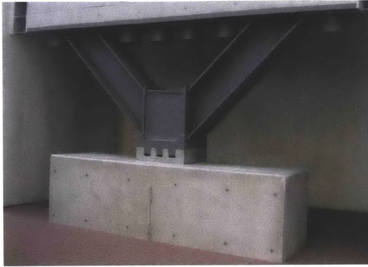
Figure 6.4.1. Open cast pin (photograph courtesy Prof. Simon Laflamme)
