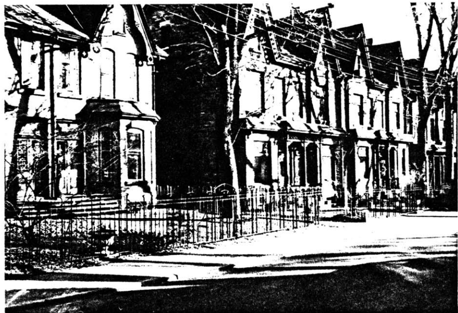
Renovated houses on Metcalfe Street.
