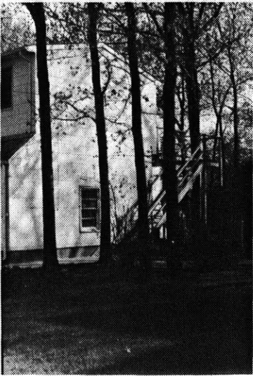
LINCENHURST, NY AN UNPAINTED, EXPOSED STAIR ACCESSES THE UPPER FLOOR OF A LOFT THROUGH A FULL DORMER.
