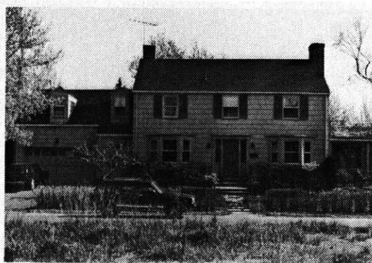
TWO-LEVEL COLONIAL, OLD GREENWICH, CT HERE BOTH FRONT AND BACK DOORS ARE VISIBLE FROM THE STREET, YET THE PROMINENT CENTRAL LOCATION OF THE MAIN ENTRY CLEARLY DIS- GUISES IT FROM THE REAR DOOR JUST TO THE RIGHT OF THE GARAGE. THE BACK DOOR COULD SERVE AS AN ENTRY TO AN ACCESSORY UNIT LOCATED ABOVE THE GARAGE.
