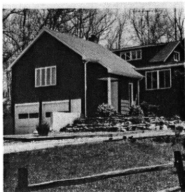
WESTON, CT AN OVER-THE-GARAGE APARTMENT WITH AN INTERNAL STAIR. NOTE ALSO THE PRIVACY OF THE SECOND ENTRY, ACCESSIBLE DIRECTLY FROM THE DRIVEWAY.
