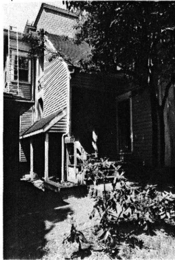
CAMBRIDGE, MA A PARTIALLY-EXPOSED STAIR IS EN- CLOSED WITH CLAPBOARD TO BLEND WITH THE HOUSE. NOTE THE OPENING AT THE TOP OF THE LANDING WHICH PROVIDES LIGHT AT THE ENTRY; ALSO THE STORAGE AREA UNDER THE STAIR.
