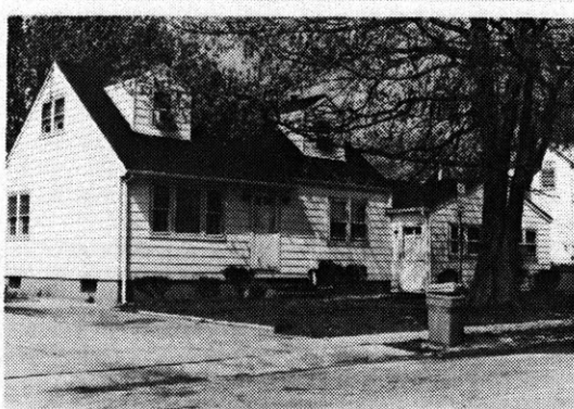
ONE-AND-A-HALF- LEVEL CAPE LARCHMONT, NY HERE, THE ENTRY TO THE SECOND UNIT, ALTHOUGH IT IS PERPEN- DICULAR TO THE MAIN ENTRY, NEVERTHELESS COMPETES WITH IT, DUE TO ITS PROXIMITY AND SIMILAR FORM.
