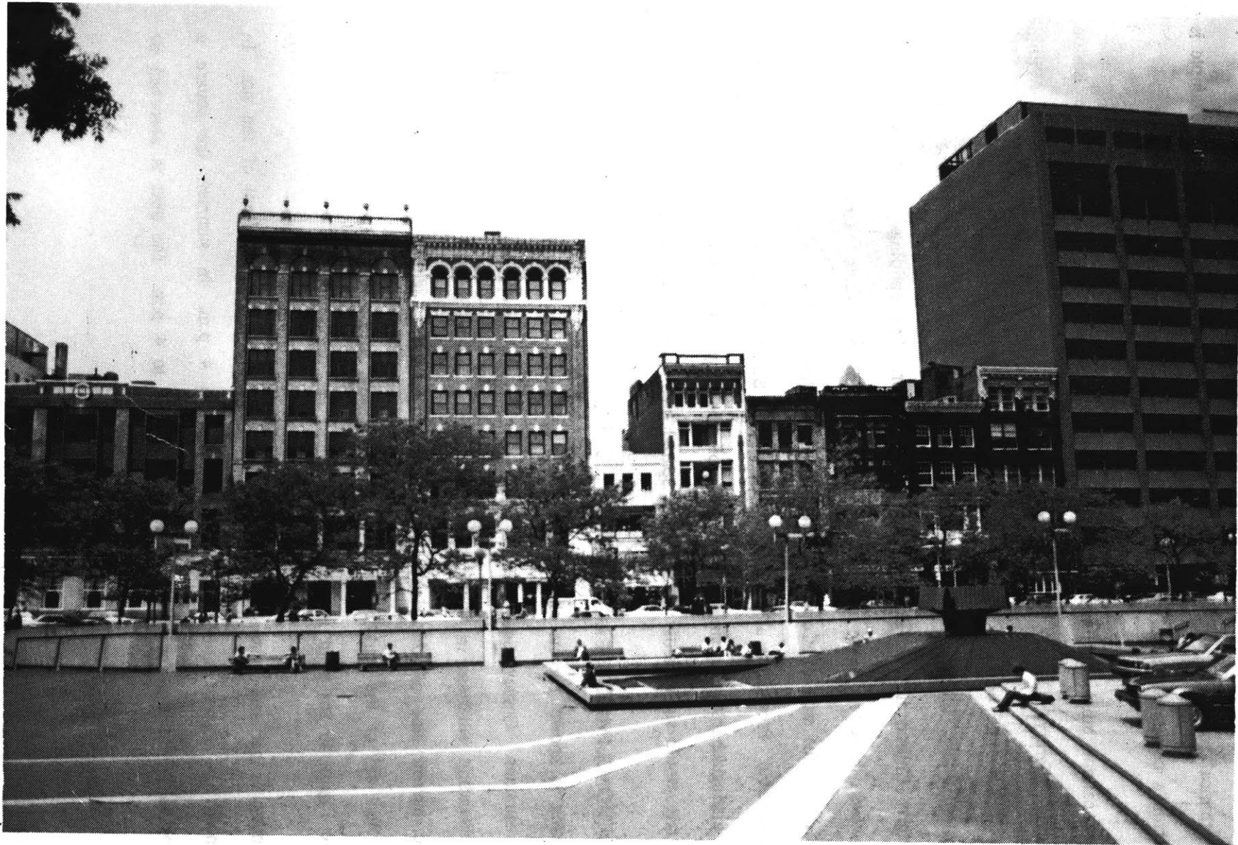
Figure 45: Facades of Boylston Street facing Copley Square, 1984.
