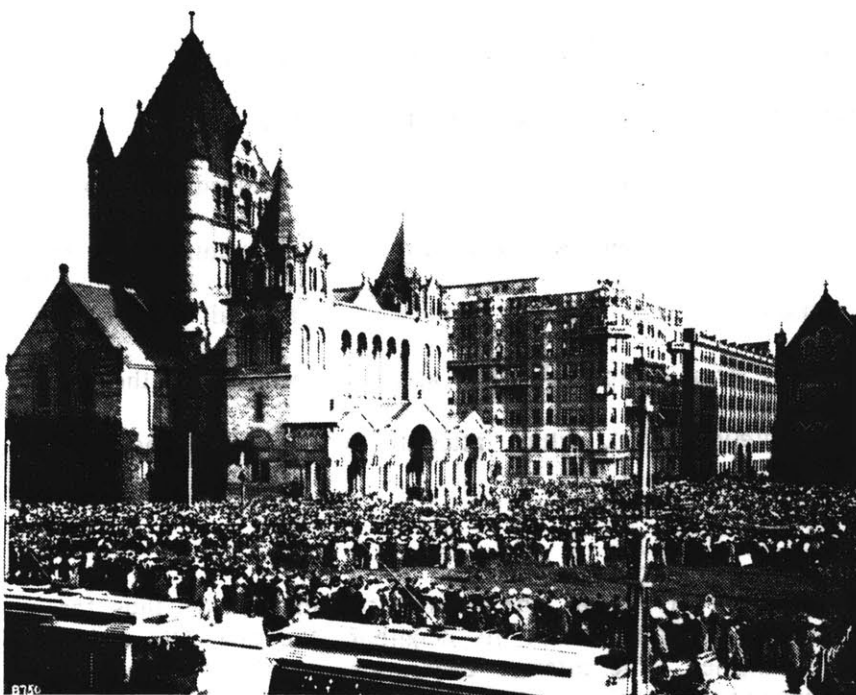
Figure 17: Trinity Church from Boylston Street, ca. 1903. Museum of Fine Arts far right, and Westminster Chambers in the middle.
