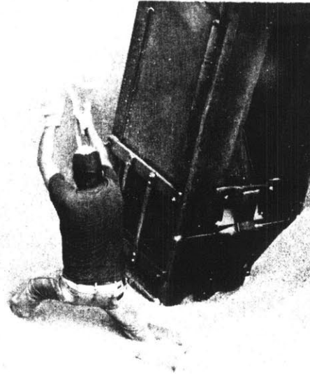
Scooper rigging power for moving to elevator marine leg, hold of steamer William A. McGonagle, Kinsman Lines, Buffalo, New York, 1985
