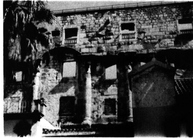
View of Roman wall at the water edge
