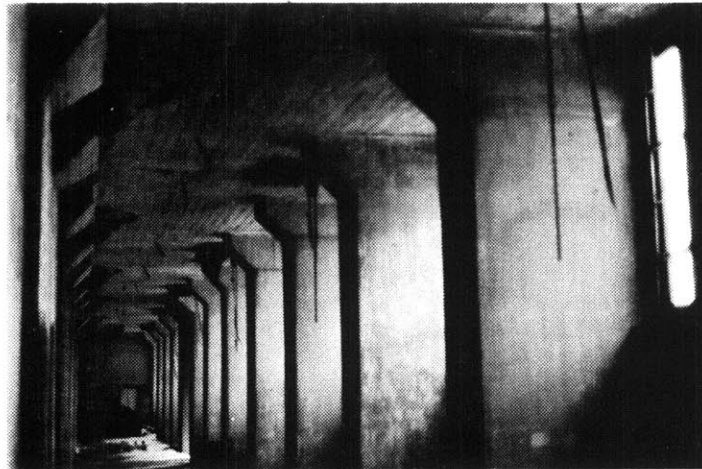
"Sea" of columns at ground level
