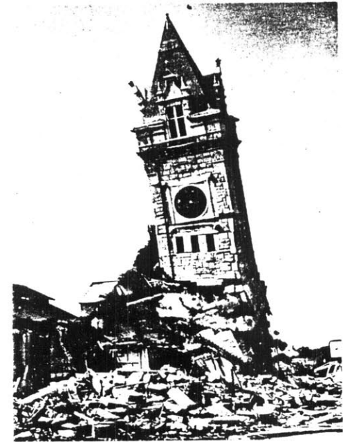
Demolition of Union station tower, Portland, OR, 1961
