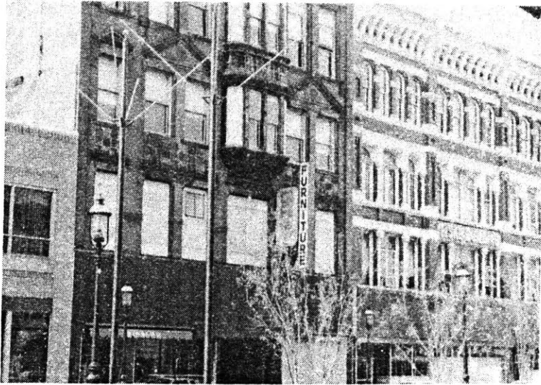
Gray and Fiske Buildings, Central Street.
