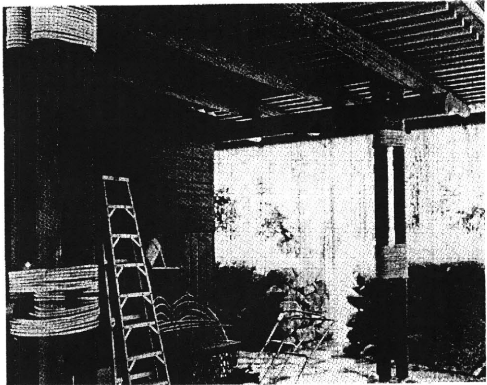
Aalto's columns at the bath house / sauna, Villa Mairea.
