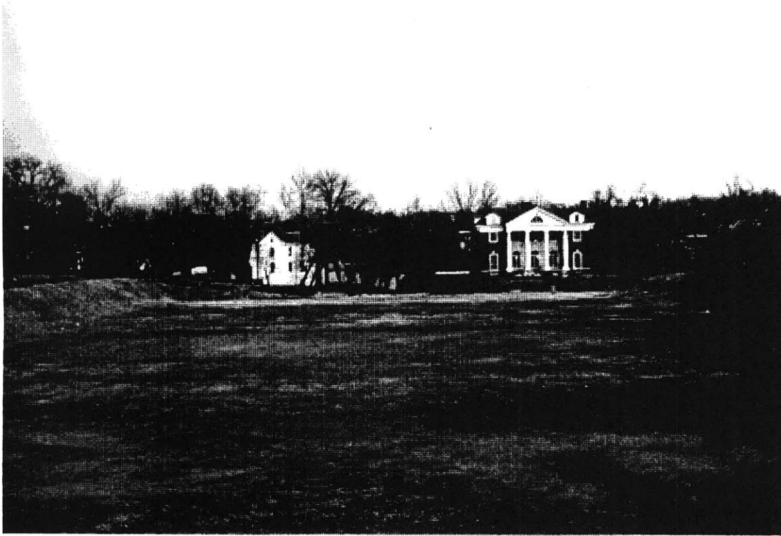
View into the site along Jeffersons axis.
