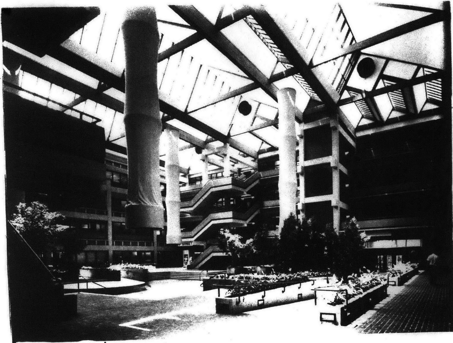
Fig.3b. The Bateson Building: Central Atrium
