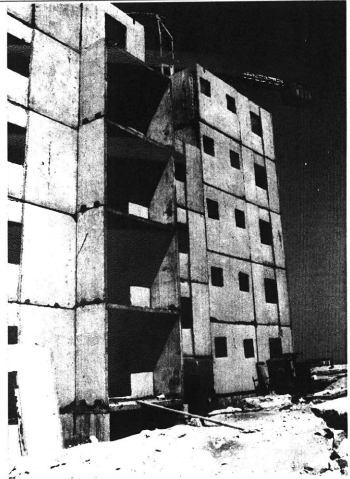
Figs. 9&10 Prefabricated housing buildings under construction near Cairo
