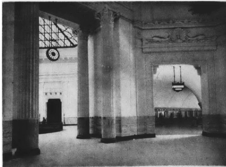
A Corner of the Foyer Hall
