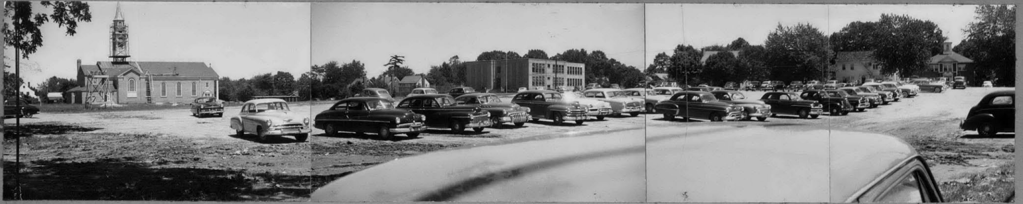
UPPER ARMORY LOT
