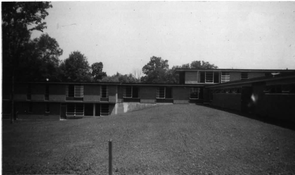
New Pre-School Nursery Unit American School West Hartford, Conn.
