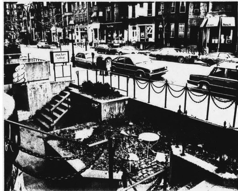
ENTRY TO BASEMENT LEVEL SHOP
