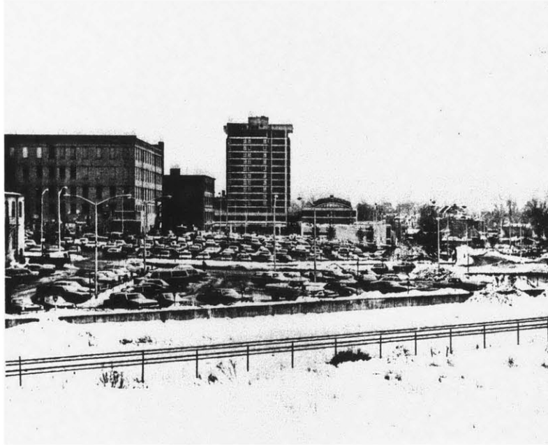
VIEW OF PARKING LOT on SITE
