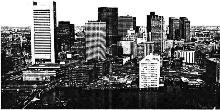
4-31 Boston skyline with Federal Reserve Bank to left.
