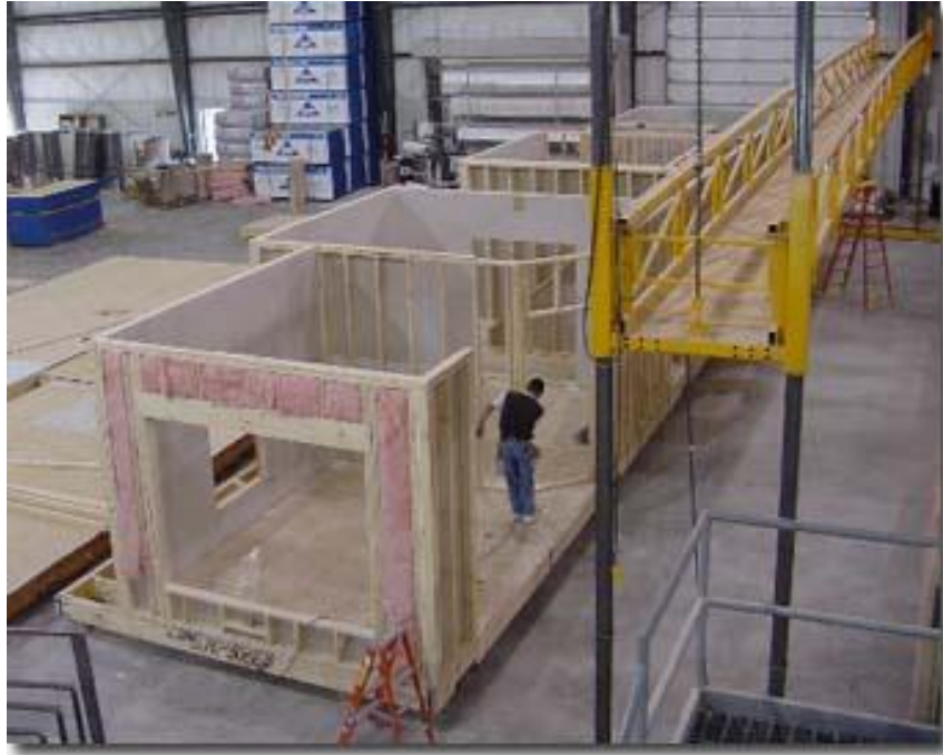
Picture 3 Insulation Prior to Exterior Finishes - Wood Frame Module
