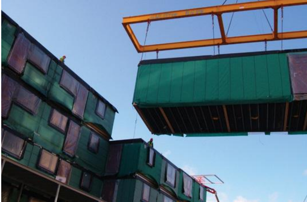
Picture 6 Steel Module Being Set
