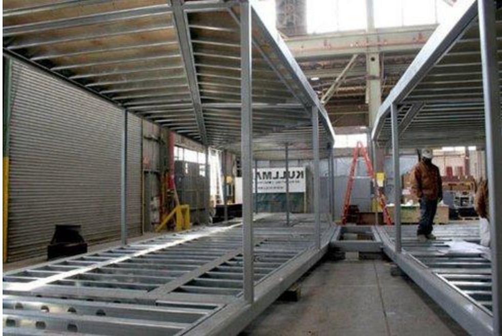
Picture 2 Typical Steel Frame Assembly
