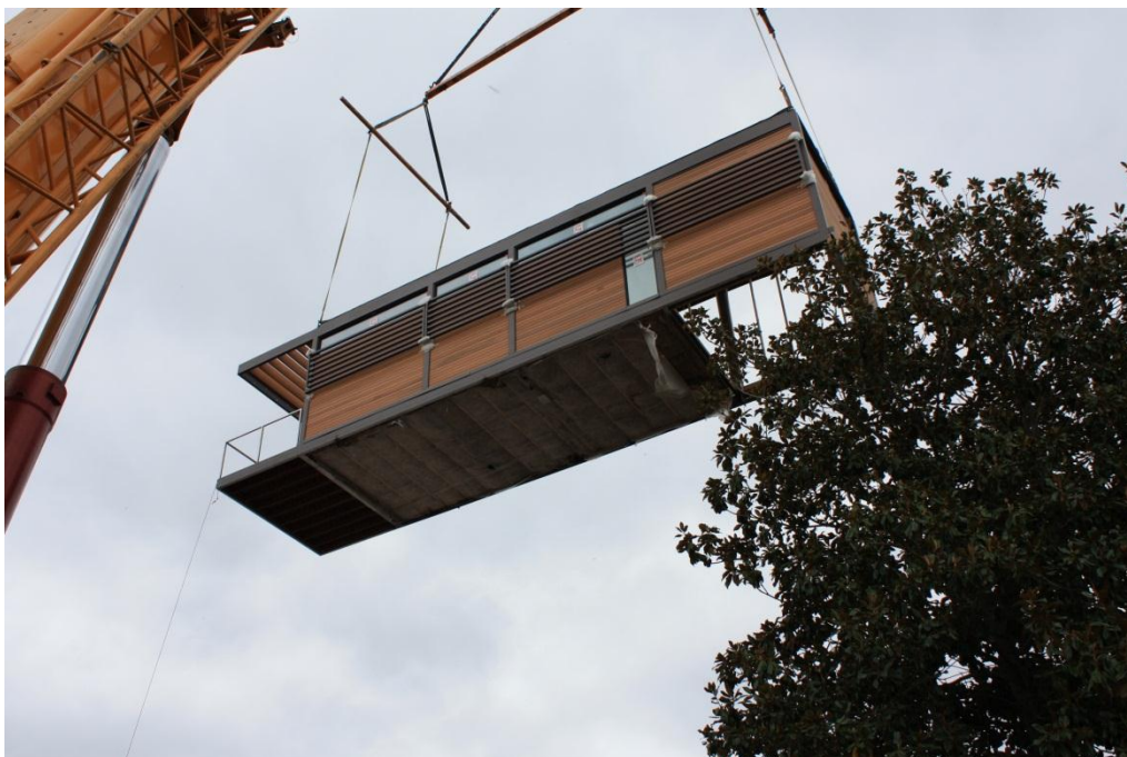
Picture 5 Lift of Steel Frame Module with Exterior Finishes
