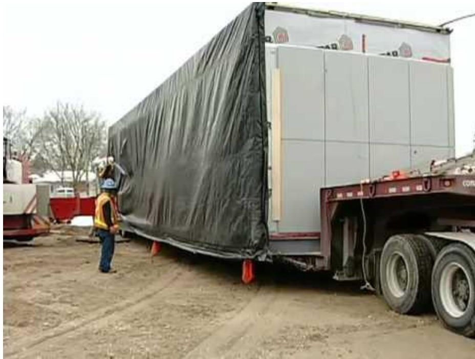
Picture 4 Flatbed Module Transport
