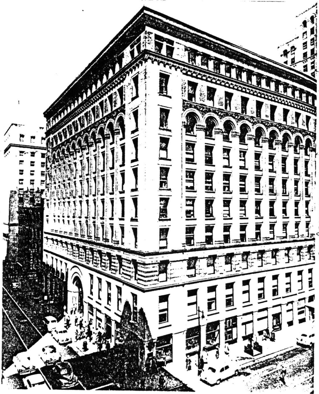
Mills Building, northeast corner of Montgomery and Bush, San Francisco,
