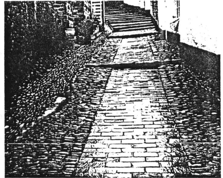
(Above and left) a steep hill visually lessened in gradient by a combination of materials and gently sweeping slopes (Minehead, Somerset, England)
