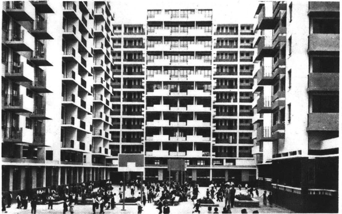
A play ground in the North Point Estate
