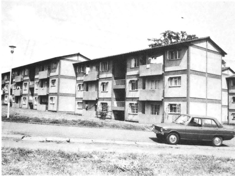
TOP, LEFT: Bukoto rental housing project. A walk-up apartment project by the National Housing Corporation for government civil servants.
