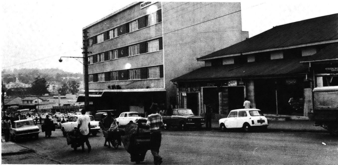
Market Street overlooking Nakivubo Car-park and Old Kampala Hill. 19th. Century Asian-type shopfronts still survive along side walk-up and high-rise concrete office blocks. Peddlers carry merchandise on hand-carts to and from Nakasero Market and Nakivubo carpark.
