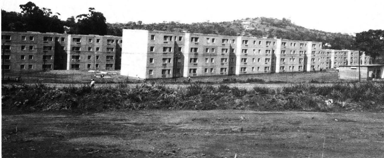
Completed stage one of Bugolobi Prefabricated Scheme; a concrete pannel experimental project. Mbuya and Kireka Hills - high income localities - in the background.
