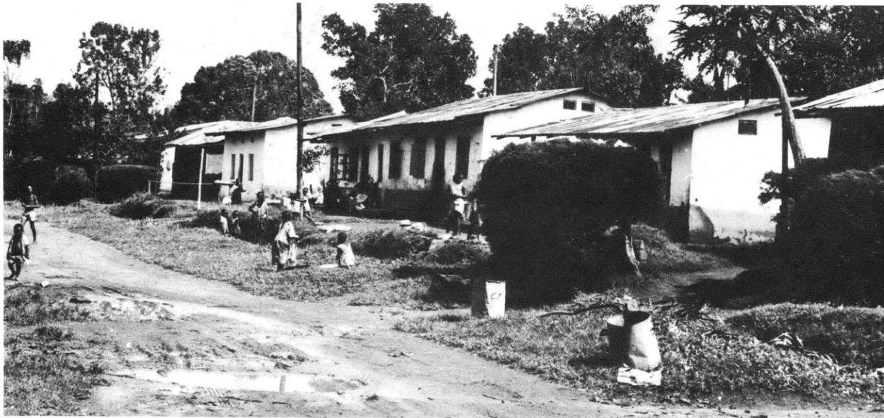
Streicher Road: Site and service Self-help Scheme. Mud/wattle houses. Murram finished roads get muddy during the rainy season and dusty during the dry season. Note children playing in storm-water trenches due to lack of sufficiently defined children play-grounds.
