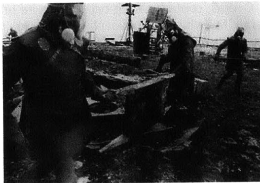
Figure 7: Local nuclear externalities | liquidators removing the highly contaminated remains of the reactor explosion
