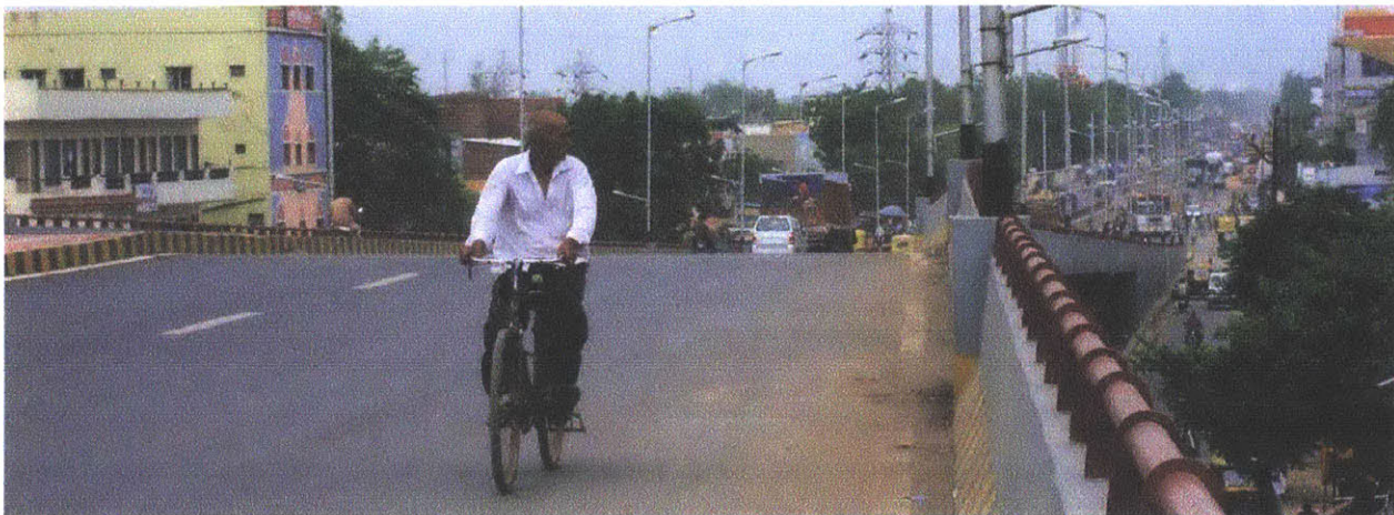
Figure 5: Newly built elevated overpass and bicyclist, Ahmedabad
