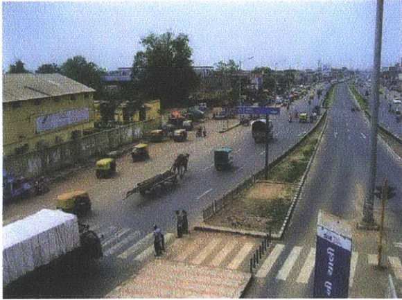
Figure 24: Narol Naroda Road - NH 8 / Corridor Survey
