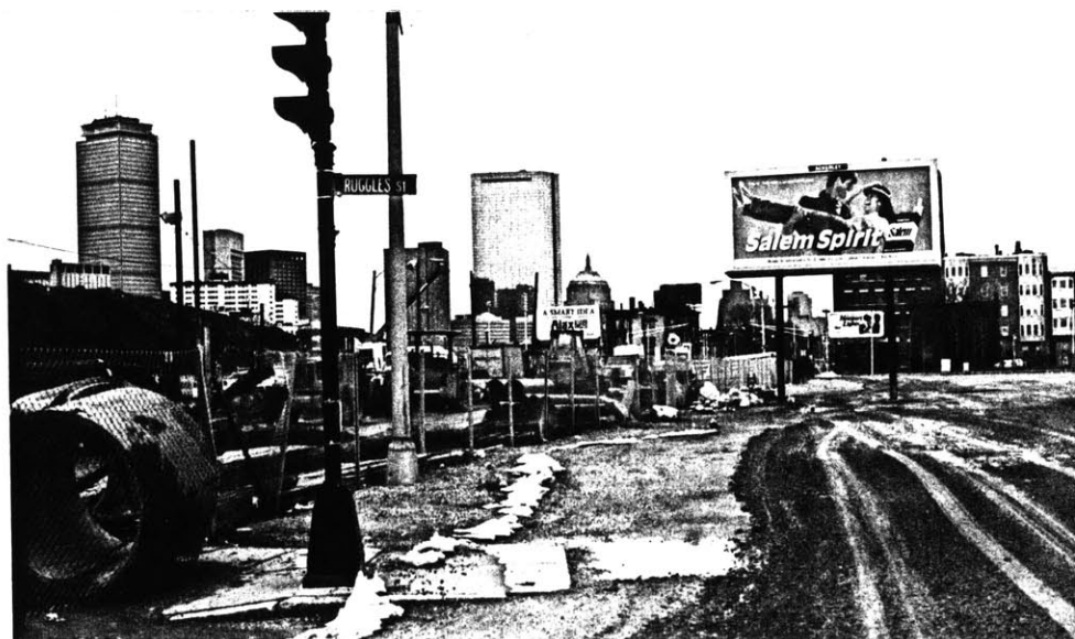
View of site looking east showing former Ruggles Street corner.
