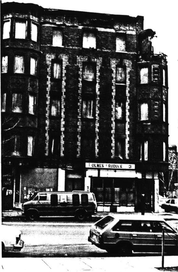
Above: Existing urban fabric in disrepair along Tremont Street
