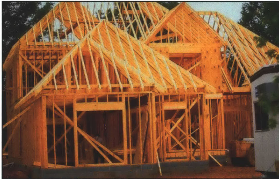
Figure 85. A typical wood frame construction of a residential building. Image source: New Home Construction
