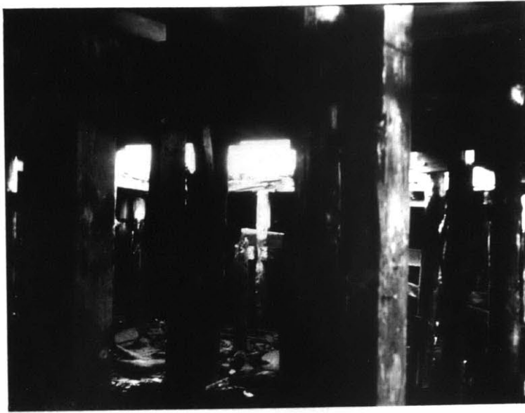
Below the same pier.
