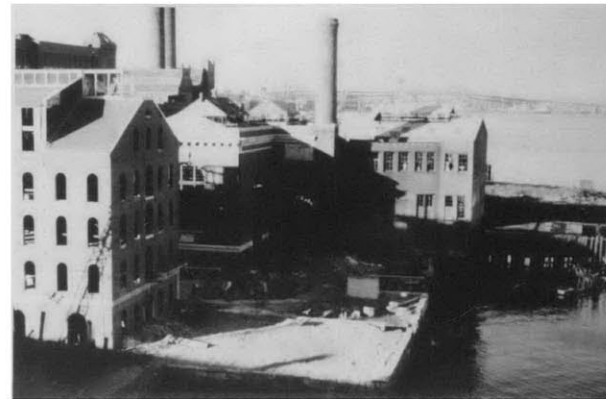
The Pilot House in the foreground, and the Generating Station. Boston, Waterfront
