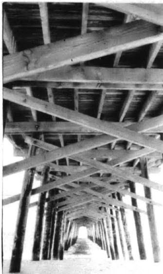
Below the same pier.
