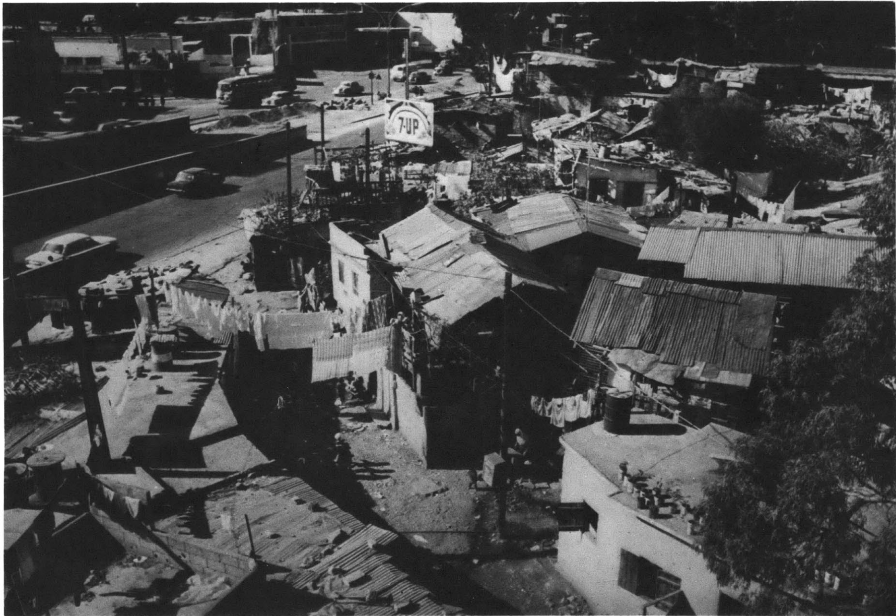
A VIEW OF THE QUARANTAINE SQUATTER SETTLEMENT In the background, the Eastern entrance of Beirut. In the foreground, the semi-rural squatter settlements occupying inner-city land of high and rising commercial value. Notice their huts made out of concrete block walls and galvanized iron sheets roofs. The settlement is located approximately two kilometers from the center of Beirut.
