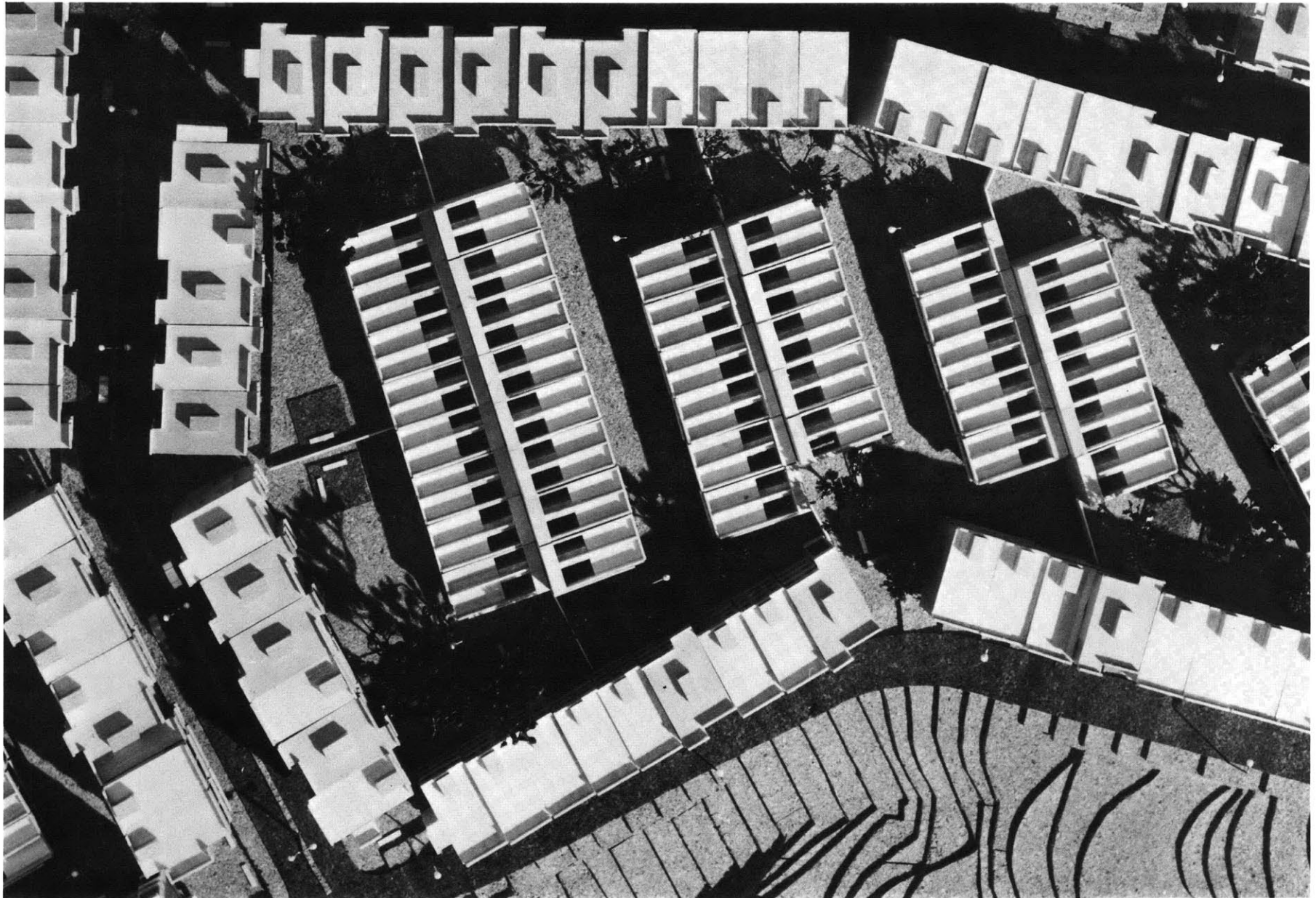
CLUSTERS ( AHIA' ) The picture shows a series of lot clusters, each containing a semi-private interior court ( SEHAT ) bounded by row houses and walk-up apartments. This interior court provides access to the dwellings and is the place for outdoor social activities of the families living in the cluster.
