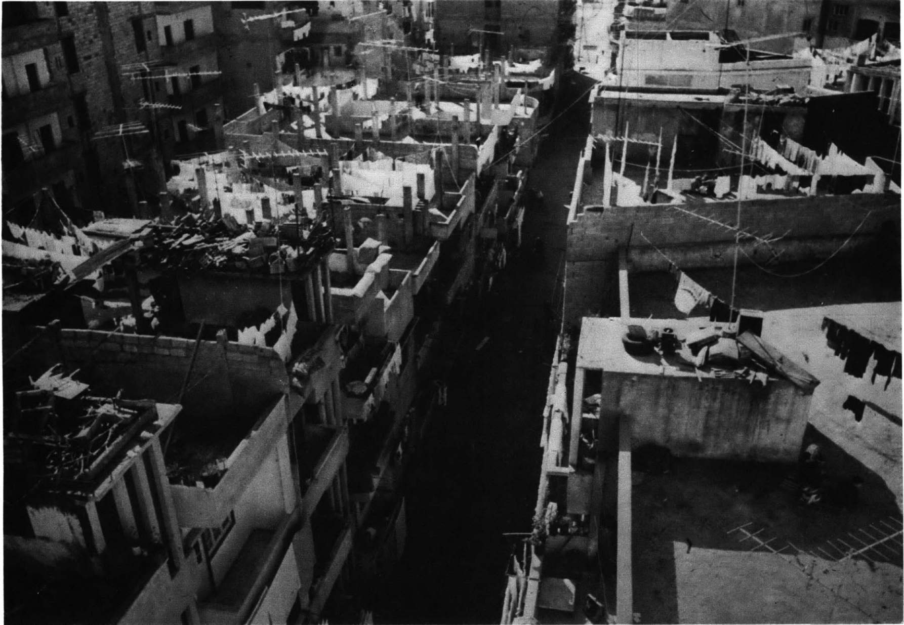
VIEW OF A STREET OF ROW HOUSES This is a typical case of illegal settlements where the houses do not comply with building codes and regulations. The plots are small, narrow and deep, sometimes built hundred percent. Notice how all the houses have been built progressively. The roofs have columns ready for future expansion, the roofs are used as recreation spaces for children, for the laundry etc. Notice the narrow streets and the very high density of population occupying this area, one of the highest in the world.
