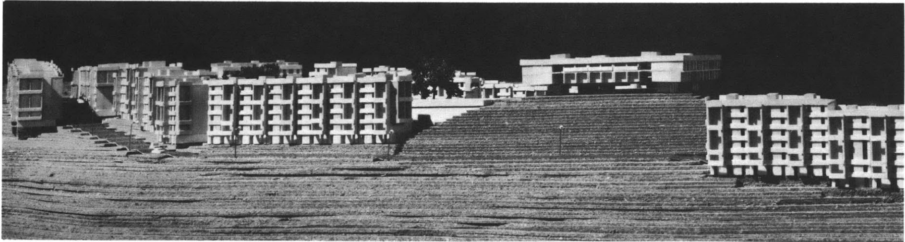
VIEW FROM THE EAST Walk-up apartments bordering the deep valley, the primary school over Tal el Mir.
