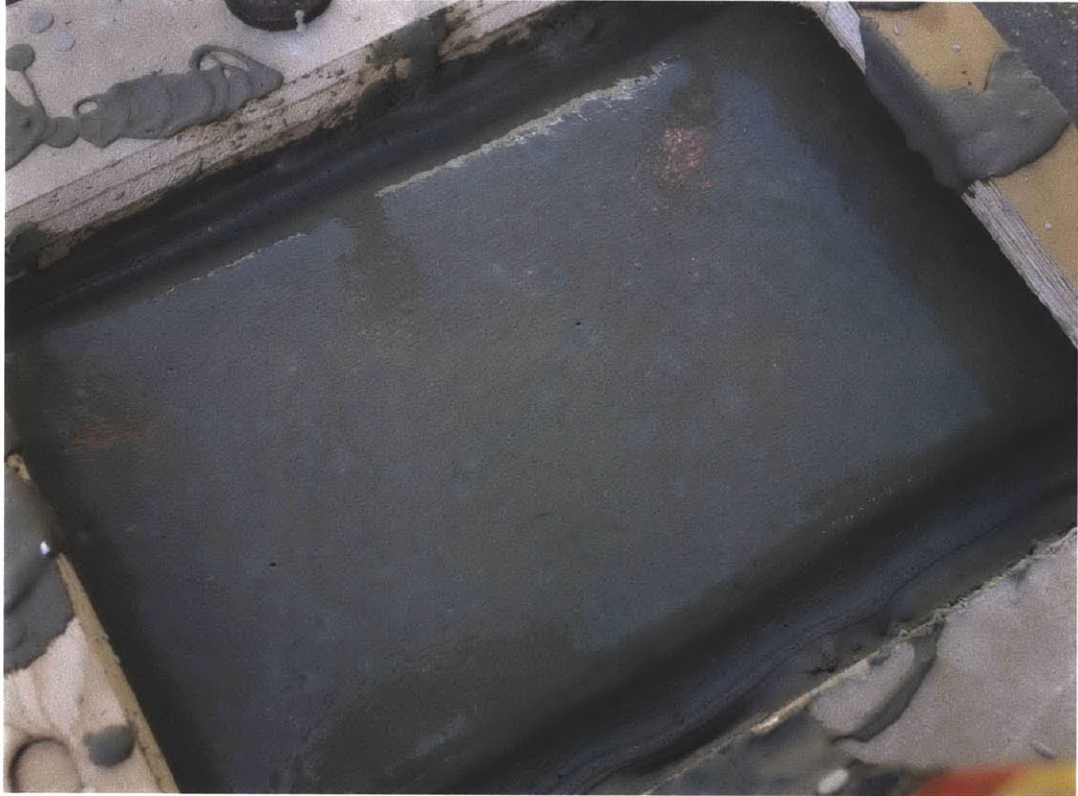
Plate 45 Close-up of expanding slurry in the gypsum beam mold
