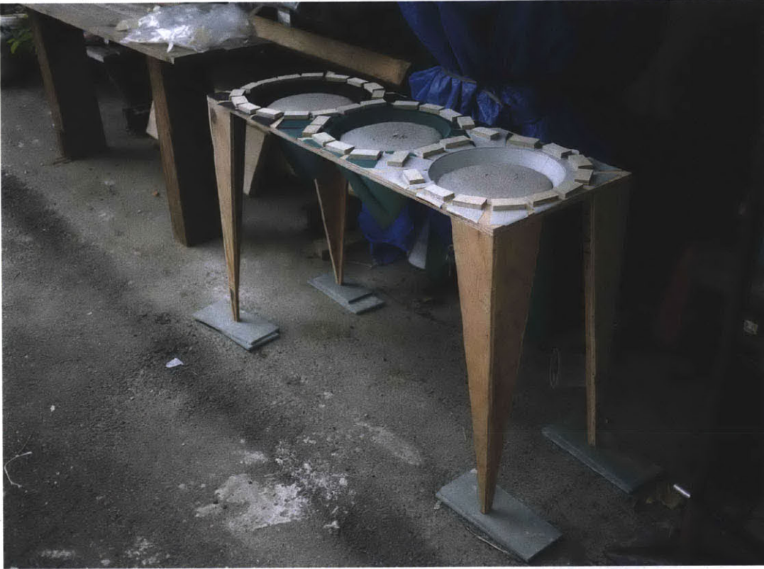
Plate 17 First round of casting in fabric molds
