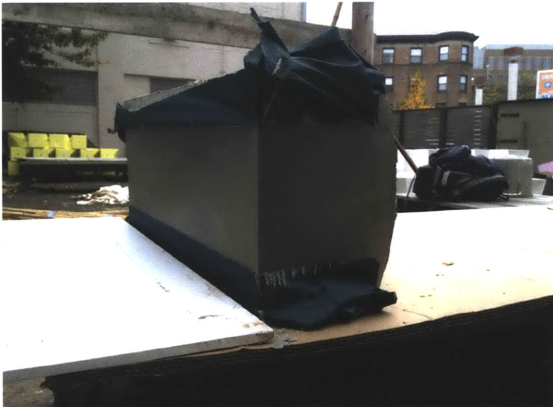
Plate 51 Second beam prototype being demolded.
